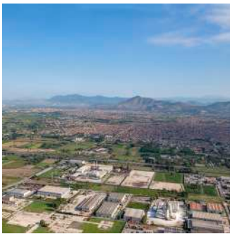
Municipality of Marcianise and a sector of the Industrial Agglomerate | Ph Paolo De Stefano, 2020
