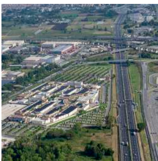
In foreground the Outlet "La Reggia" and on the left a sector of the Industrial Agglomerate | Ph Paolo De Stefano, 2020
