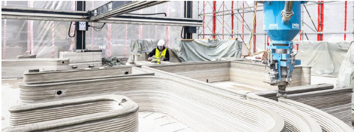
Fig 3. The HeidelbergCement research team is developing material formulations that can be used in various 3D printing techniques. Image source: GPI HC Group
