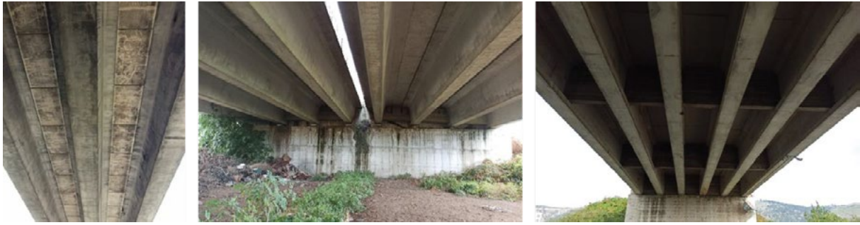
Fig 3. Typical conservation state of inspected prestressed reinforced concrete bridges.
