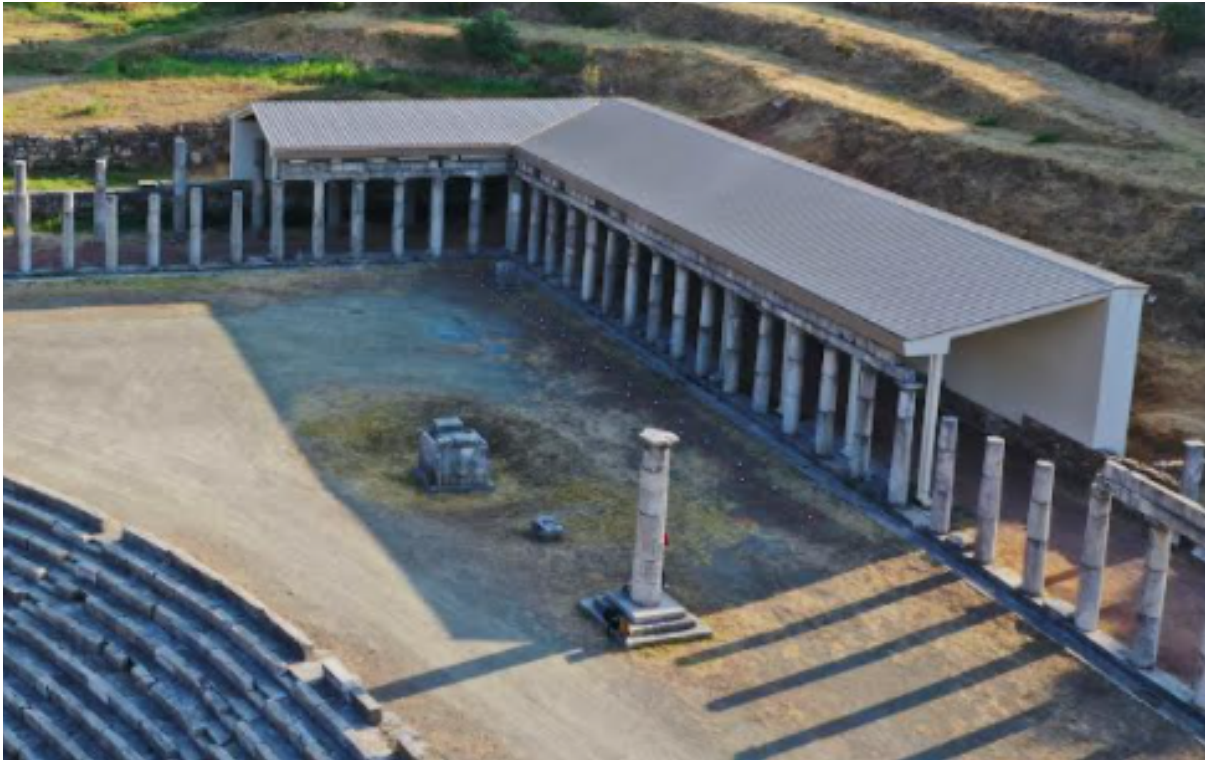
Fig 1. Messene: a view of the monument, after the intervention, where the steel columns and members are hidden behind the ancient columns and lintels
