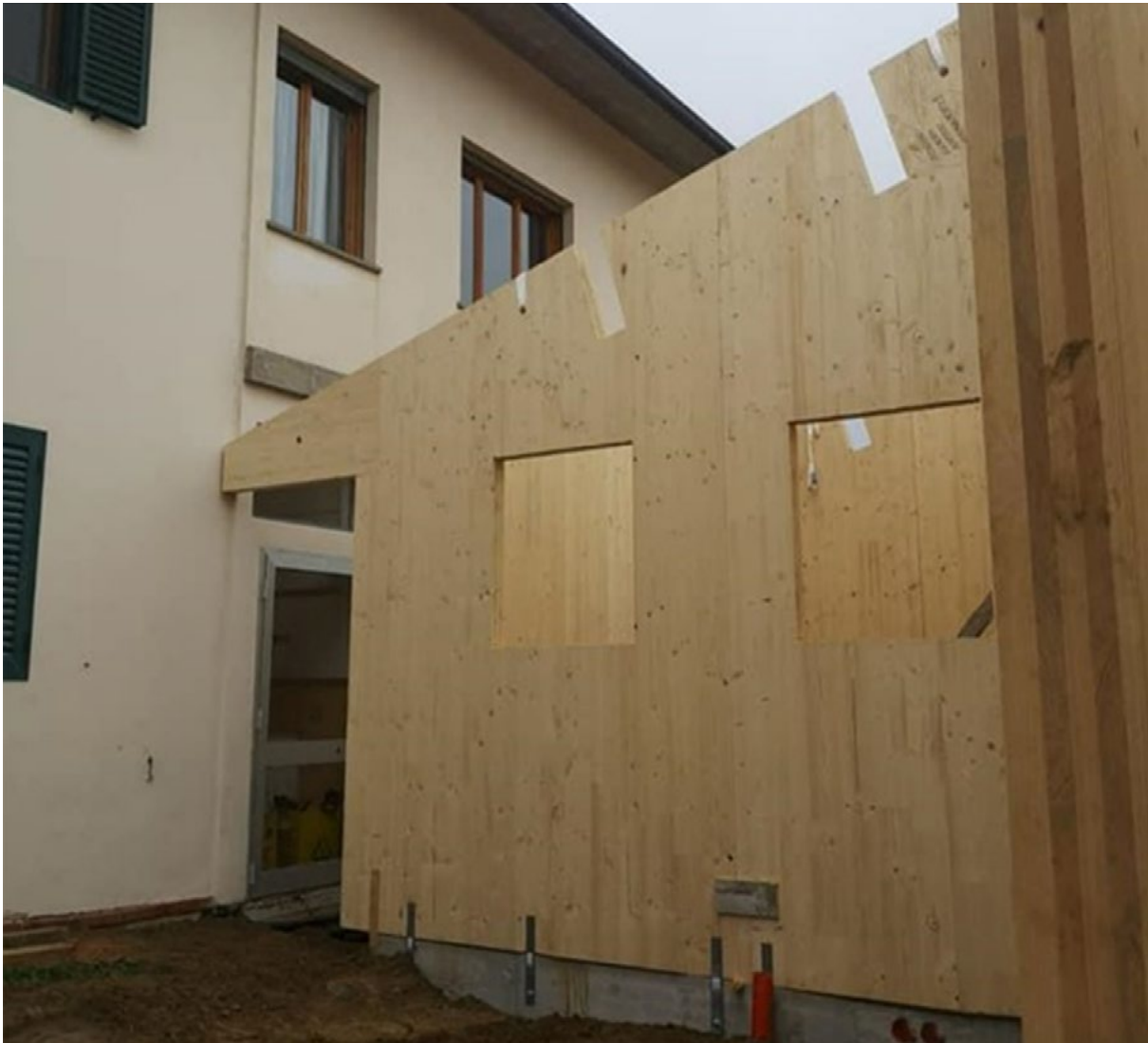
Fig. 1 CLT panel: example of installation.
