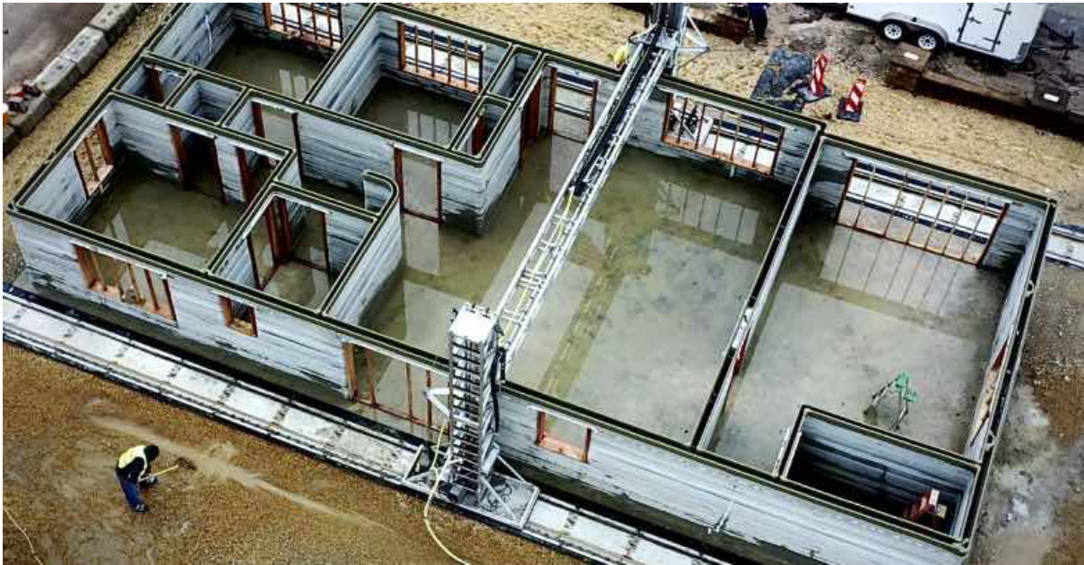
Fig 2. Construction site of 3D Autonomous Robotic Construction System (ARCS). Image source: GPI HC Group.
